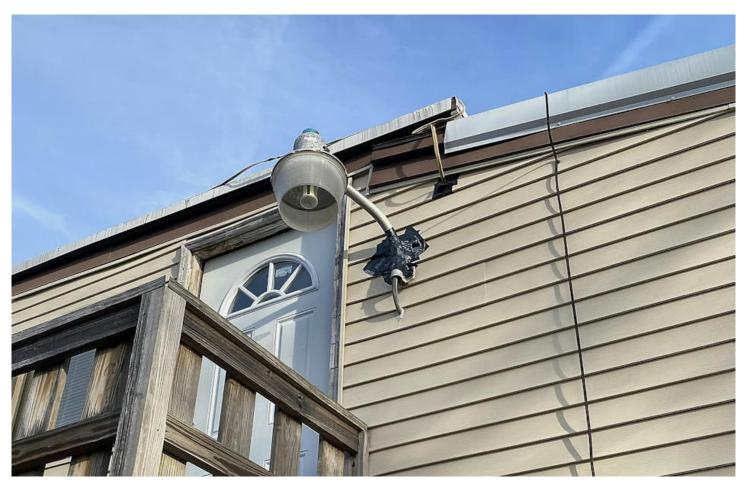
That black "blob" all over the mounting bracket of the luminaire is tape. The metal bracket is broken, and if it weren't for the tape holding everything in place, the luminaire would be dangling upside-down by the circuit wires.
